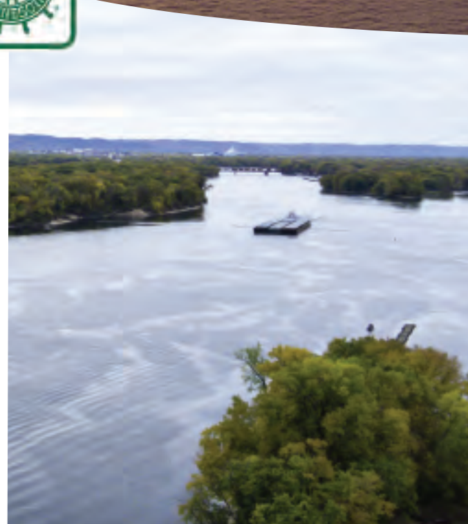
Lock And Dam #7 La Crescent Minnesota
